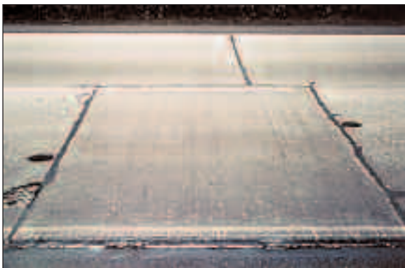
Figure 88: Distress Type JCP 15 Large, Low Severity Portland Cement Concrete Patch
