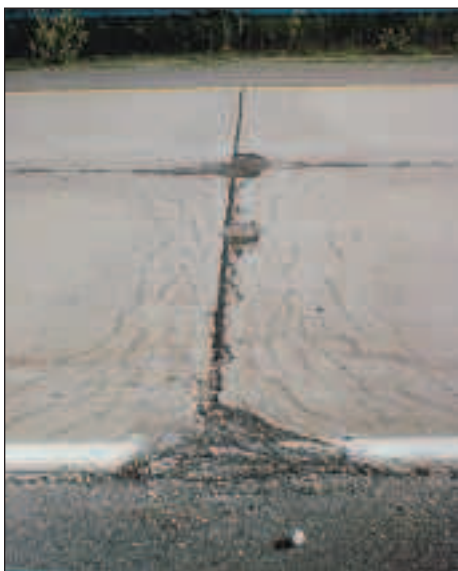
Figure 53: Distress Type JCP 2 High Severity “D” Cracking with Loose and Missing Material
