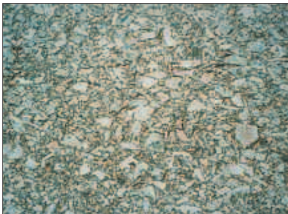
Figure 39: Distress Type ACP 12 - Polished Aggregate
