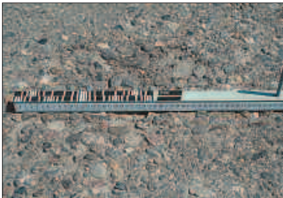
Figure 42: Distress Type ACP 13 Loss of Coarse Aggregate
