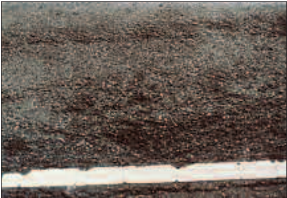
Figure 41: Distress Type ACP 13 – Moderate Severity Loss of Fine and Some Coarse Aggregate
