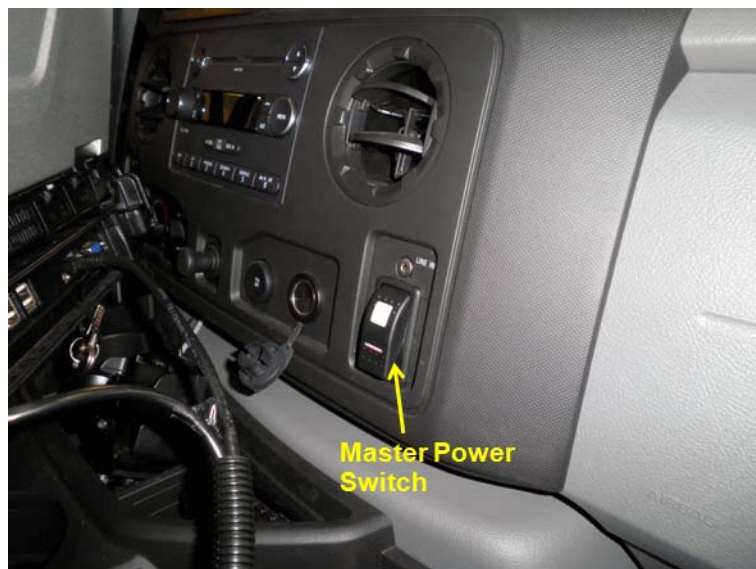
Figure 34. Master power switch.
