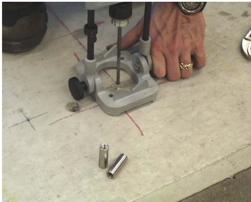
Figure 108. Photo. Concrete anchor installation step 3.
