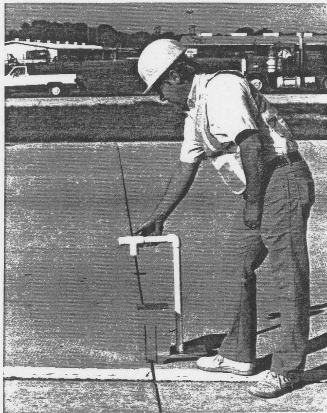
Figure 4. Operating the Faultmeter
