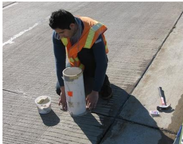
Figure 29. Photo. Infiltration Testing
