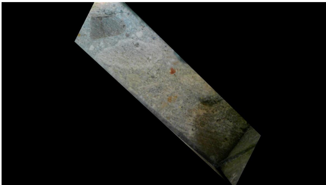
Figure 23. Photo. 1/2-inch joint face, 15 minutes after 3,500psi water blast.
