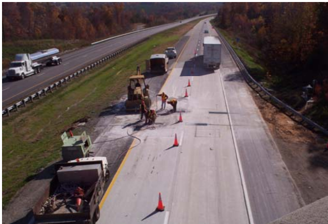
Figure 2. Pooled Fund WIM Installation on U.S. 29 near Danville, VA.
