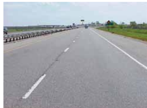
Above: A pavement test section with a 2-in. recycled asphalt overlay.
