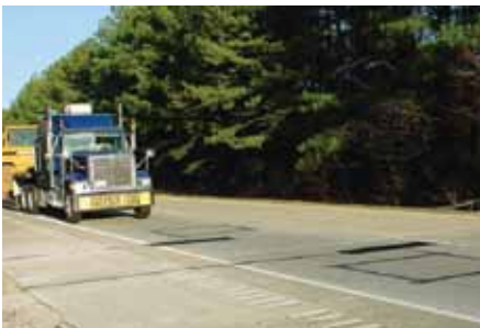
Truck approaching a WIM installation in Arkansas.
