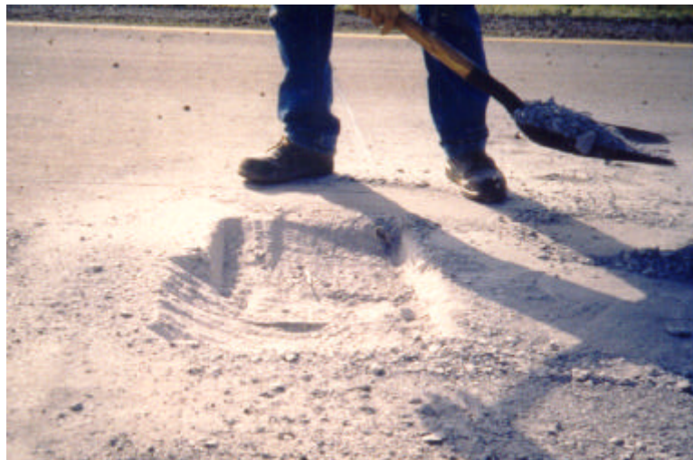
Figure 7b. Milled patch with rounded edges.
