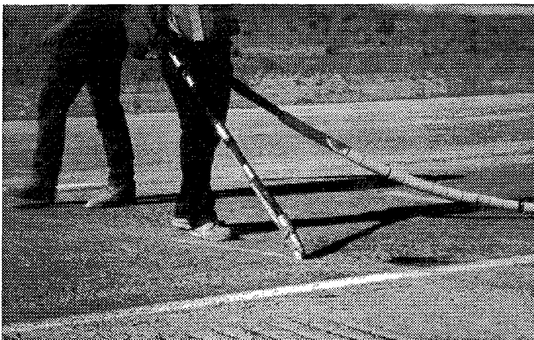
Figure 16. Sandblasting operation at Wells, Nevada test site.
