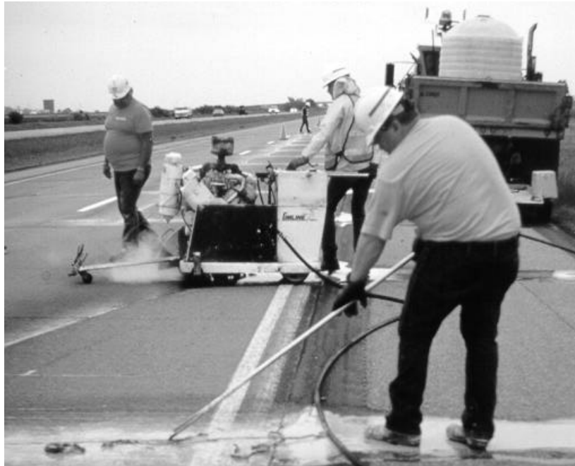
Figure 13. Joint resawing operation.
