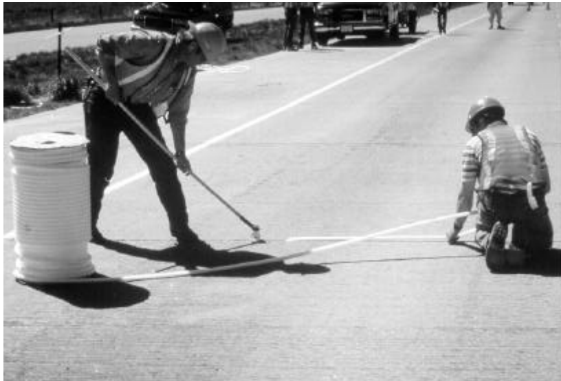
Figure 16. Backer rod installation.
