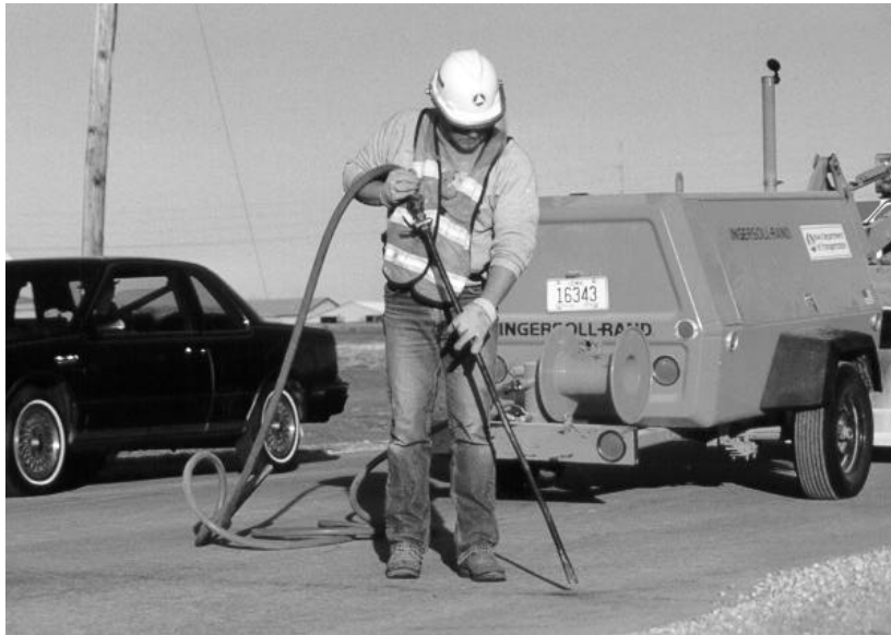
Figure 15. Airblasting operation.
