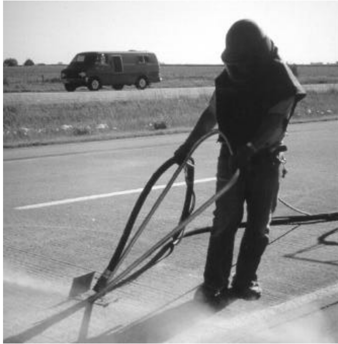
Figure 14. Abrasive blasting operation.
