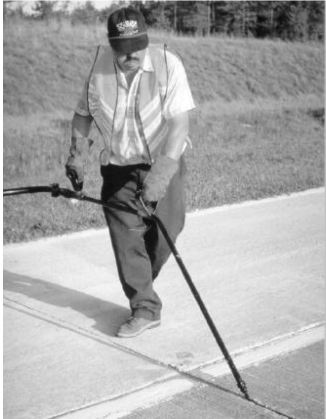
Figure 17. Hot-applied sealant installation.
