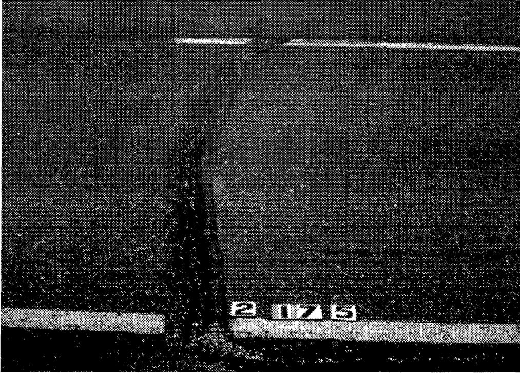
Figure 10. Hi-Spec reservoir-and-flush configuration (configuration A).
