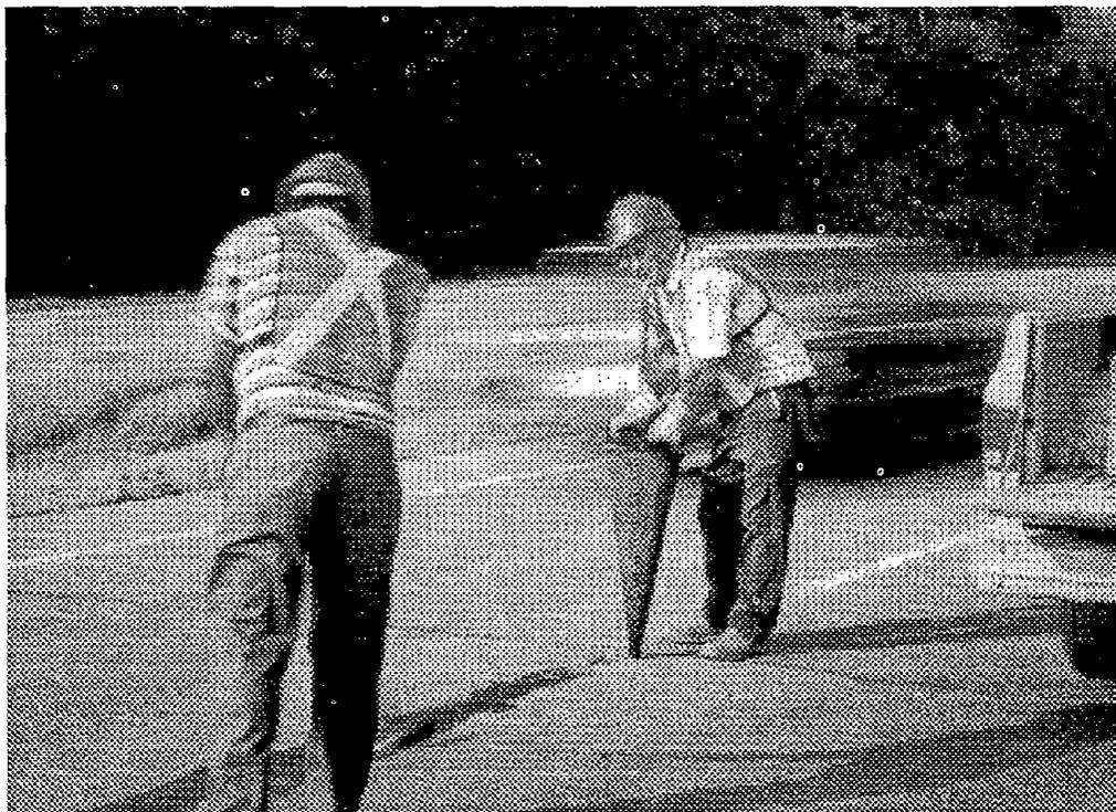
Figure 15. Placement of CRF in flush-fill configuration (configuration G).
