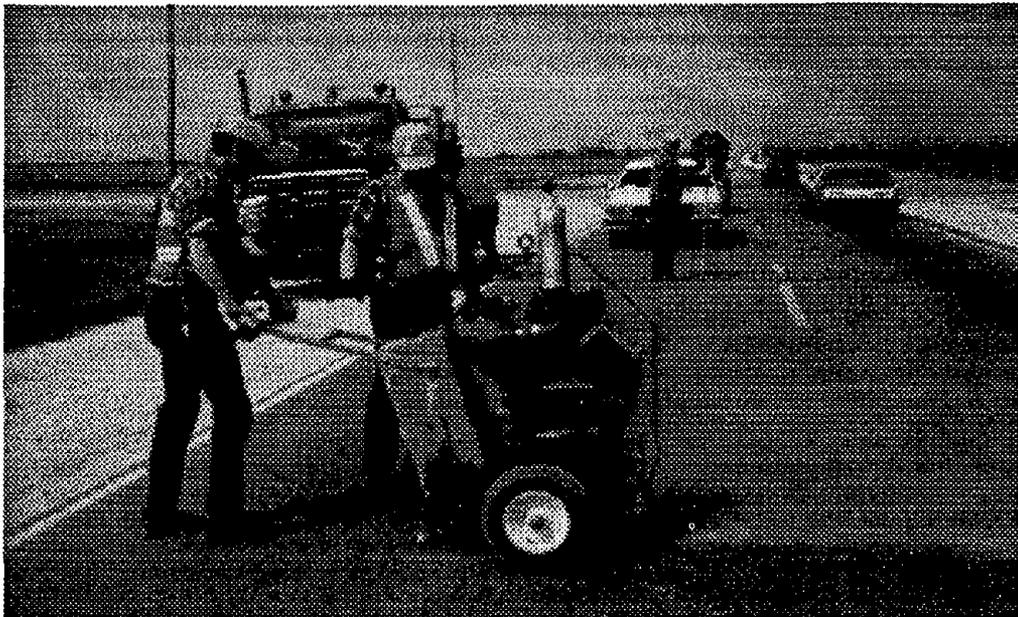
Figure 17. Random crack saw with 200-mm diamond blade.
