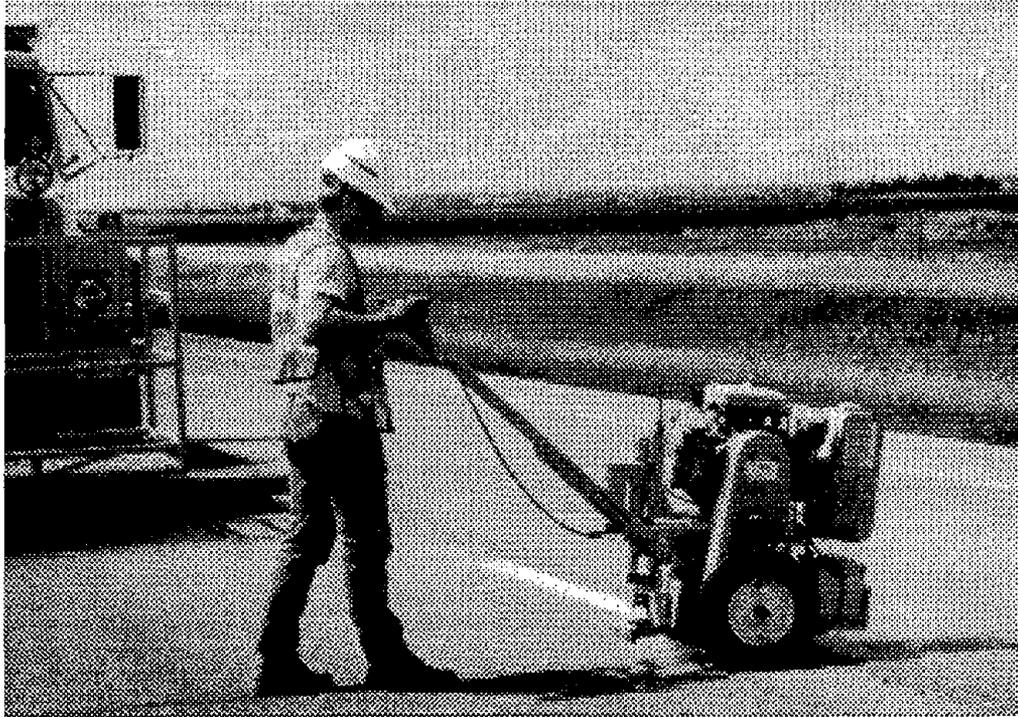
Figure 16. Carbide-tipped rotary-impact router.
