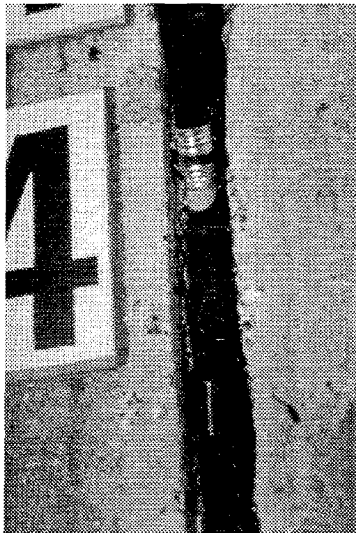
Figure 24. Partial-depth adhesion loss.
