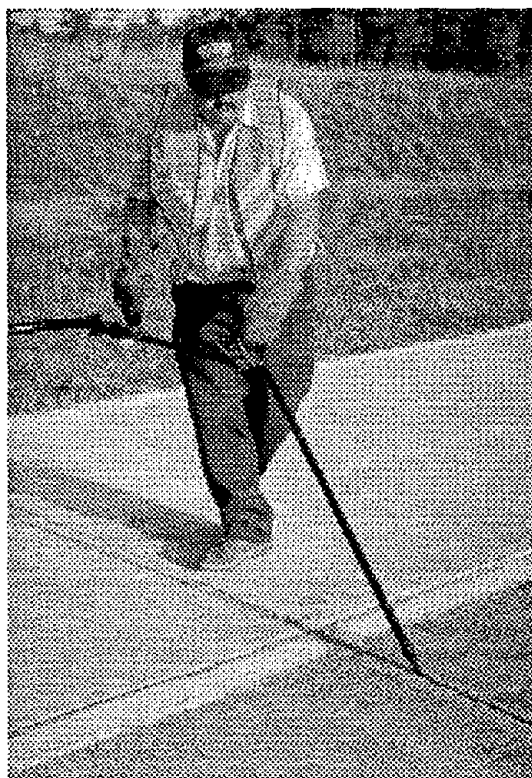
Figure 16. Recessed sealant installation.
