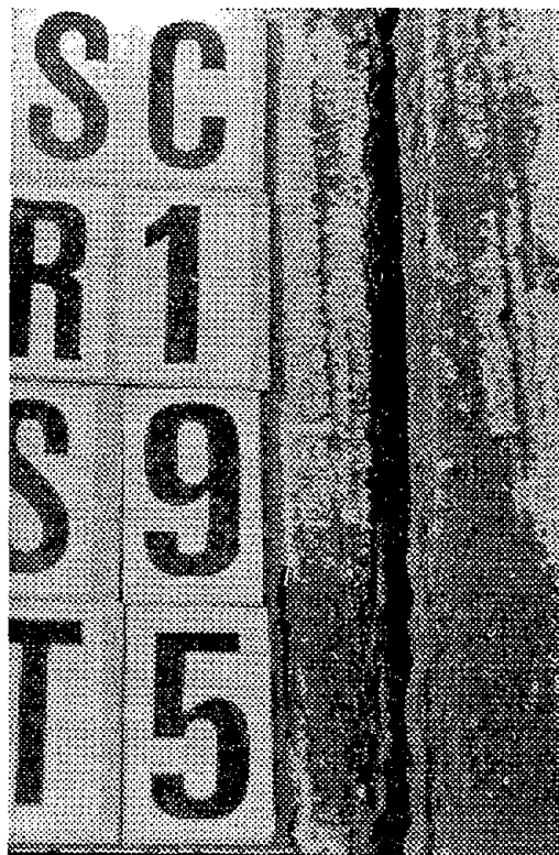
Figure 26. Overband wear.
