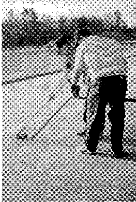
Figure 18. Overbanded sealant installation.
