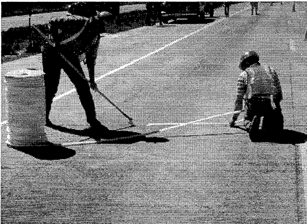
Figure 15. Backer rod installation.
