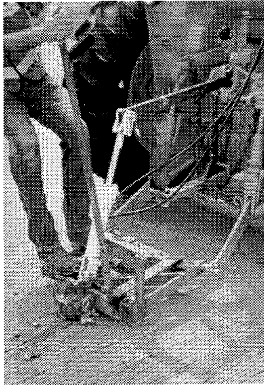
Figure 10. Joint plowing operation.
