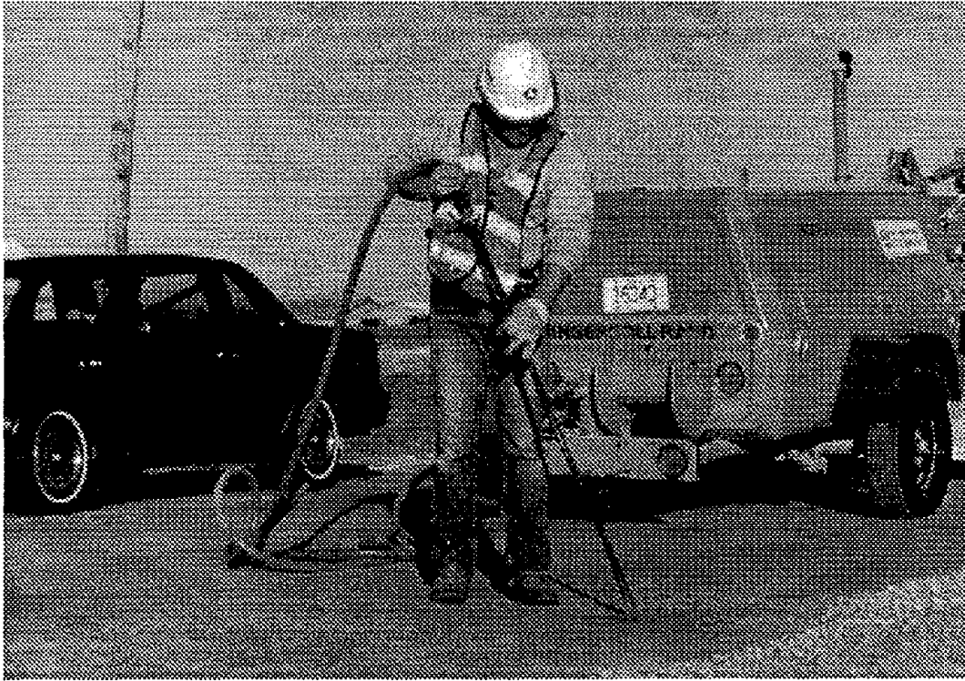
Figure 14. Airblasting operation.
