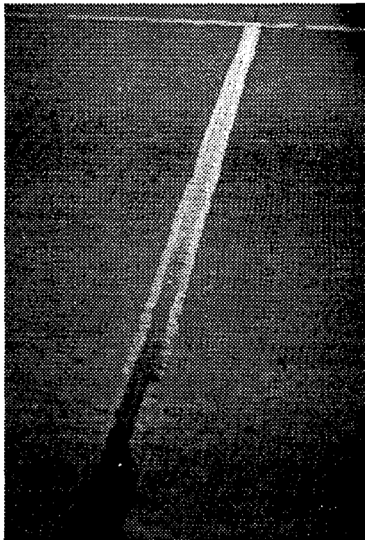
Figure 18. Overbanded sealant installation.
