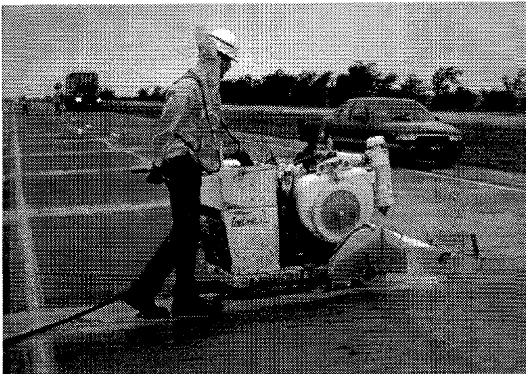
Figure 11. Joint-sawing operation.
