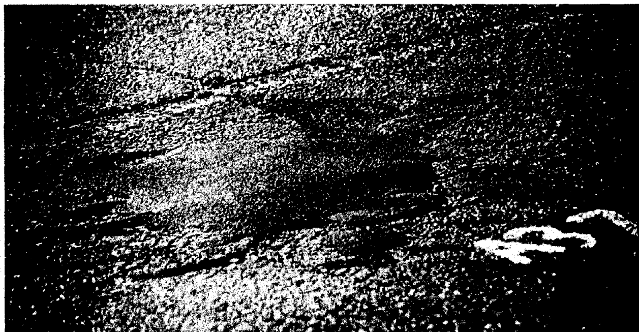
Figure 34. Example of edge disintegration distress.
