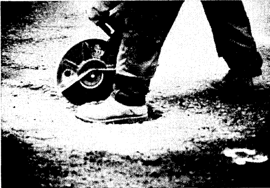
Figure 15. Straightening sides using pavement saw.
