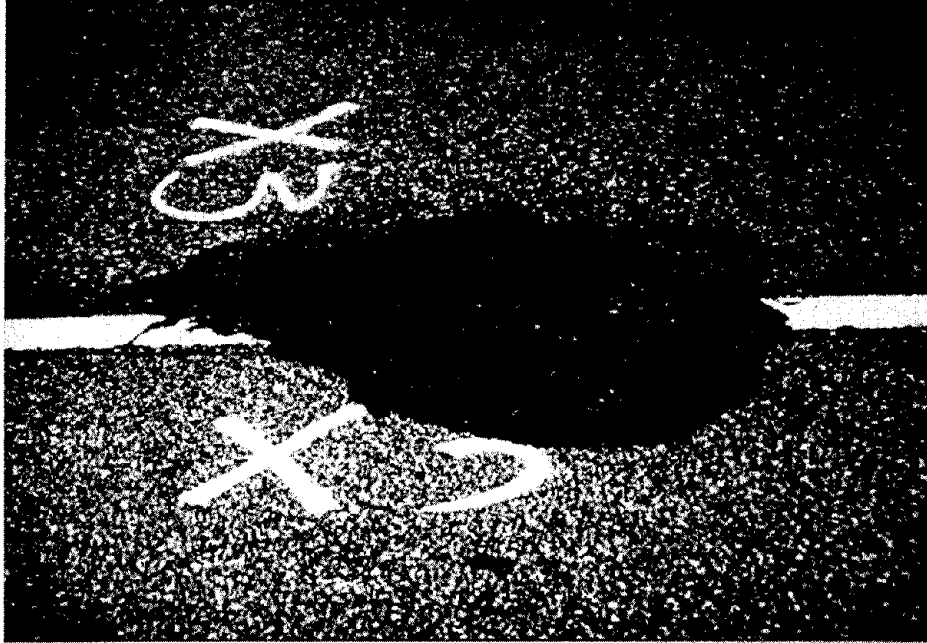
Figure 31. Example of shoving distress.
