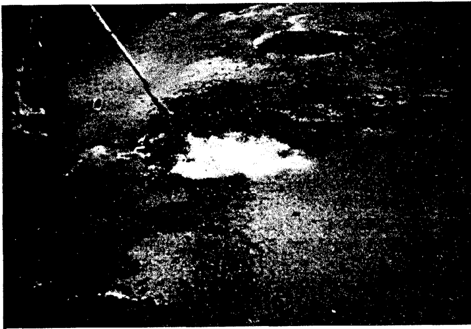
Figure 17. Heating cold mix with propane torch.
