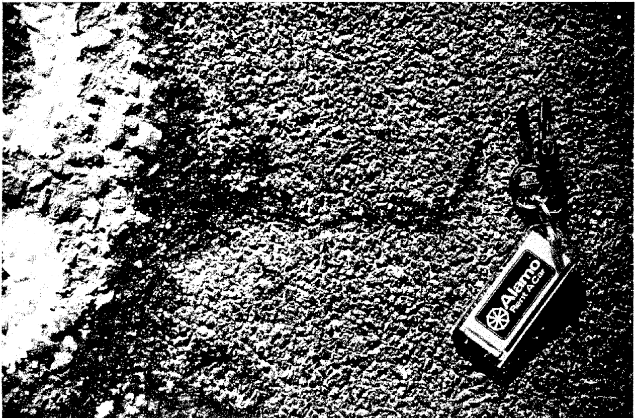
Figure 32. Example of cracking distress.
