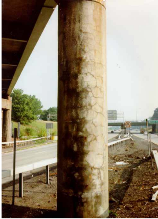
Figure 37. Photo. Cracking on the patched areas on one of the columns of the Campus Loop Bridge in Albany, NY, during the first evaluation in 1995.
