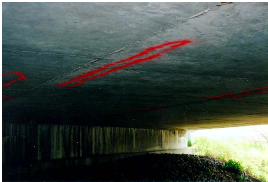
Figure 29. Photo. Delaminated areas (marked in red) on the soffit of the bridge.
