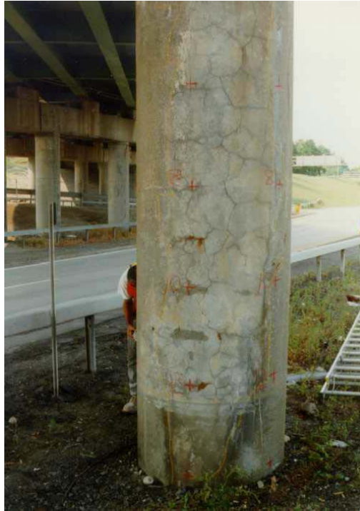
Figure 39. Photo. Second view of cracks and rust staining in patched and nonpatched areas of the columns of the Campus Loop Bridge in Albany, NY, during the second visit in 1996.
