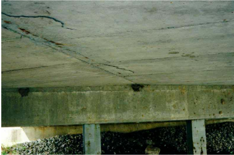
Figure 28. Photo. Cracking, rust staining, and spalling on the soffit of the bridge.
