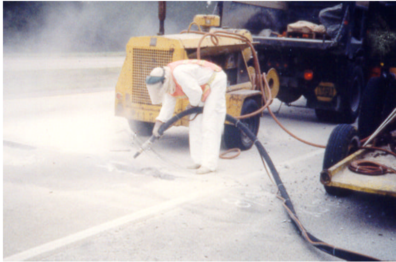
Figure 17. Sandblasting.
