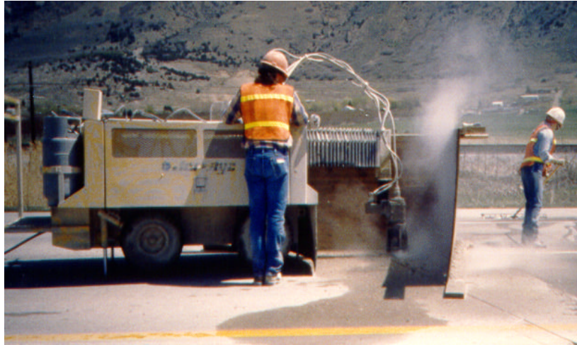
Figure 16. Protective shield around waterblasting operation.
