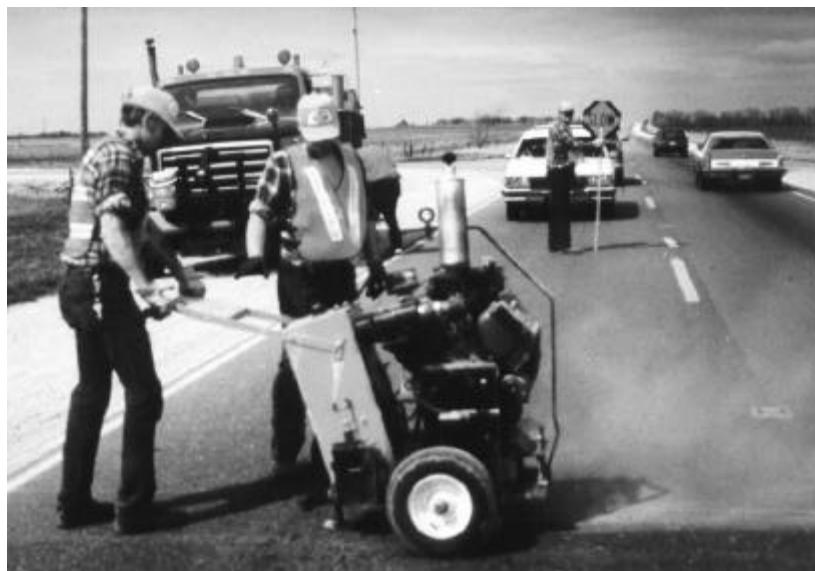
Figure 8. Diamond-blade crack saw.
