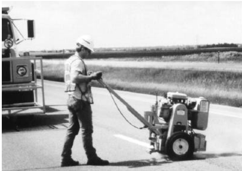
Figure 7. Rotary-impact router.
