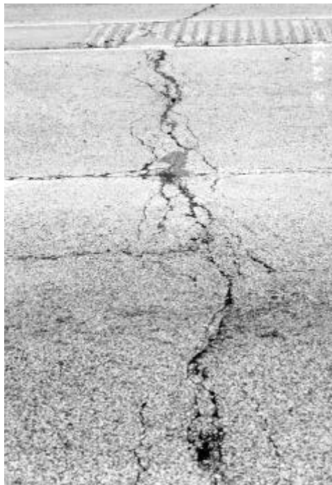
Figure 3. Pavement candidate for crack repair.
