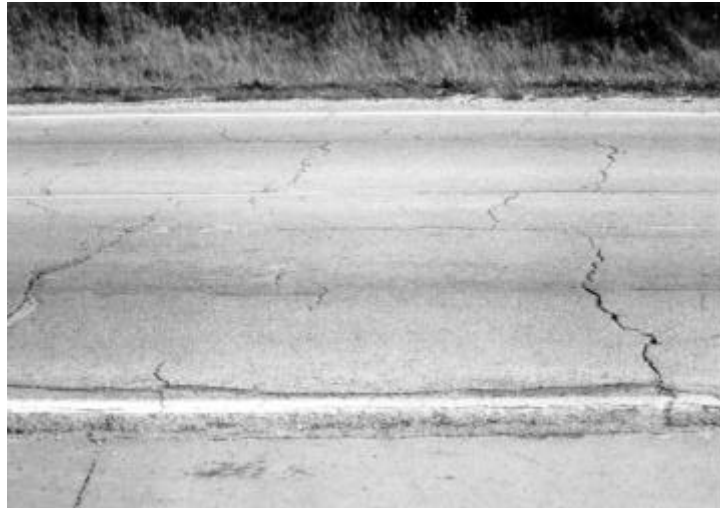
Figure 2. Pavement candidate for surface treatment: high-density cracking.
